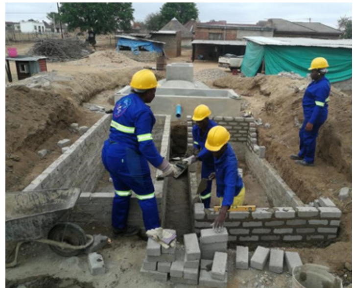
Trainees finalizing the construction of the compost pits for a twelve cubic metre digester constructed at Manjorjo Farm in Magoro
